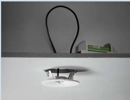
Recessed K1: connect the luminaire through the driver, install it in the ceiling and click the luminaire in place.
